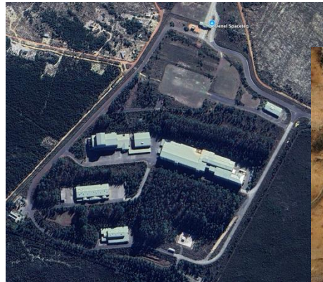
Houwteq AIT Facility
